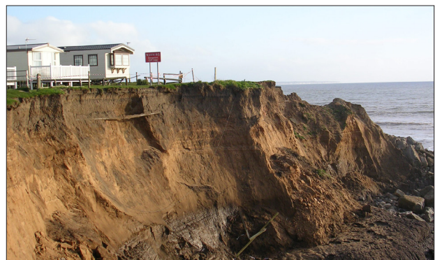
Abb.2: Kliff-Abbruch in Barmston, Yorkshire, UK (Foto: Peter Kennett)
